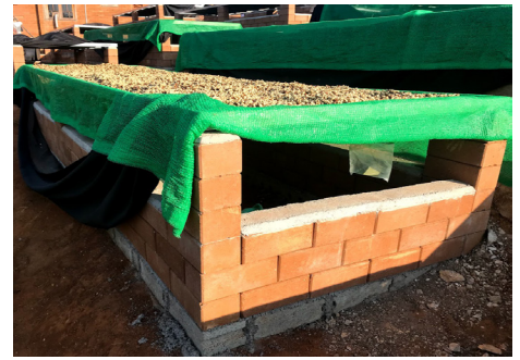
Figure 2: Raised beds constructed out compressed earth blocks, made on site.
