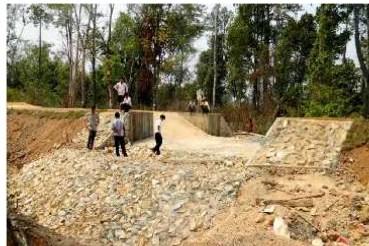
Earth dam & concrete spillway
