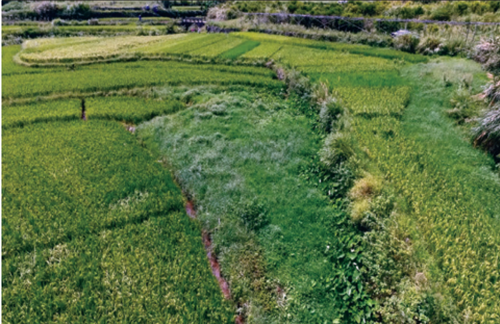
FIGURE 8.13 A bird's eye view of constructed wetlands within a rice field in Ruiyun Village*
