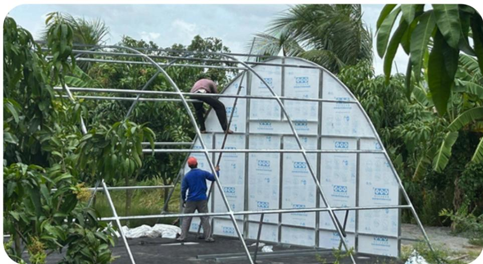
Figure 3: Bending the roof beam, CDEA
