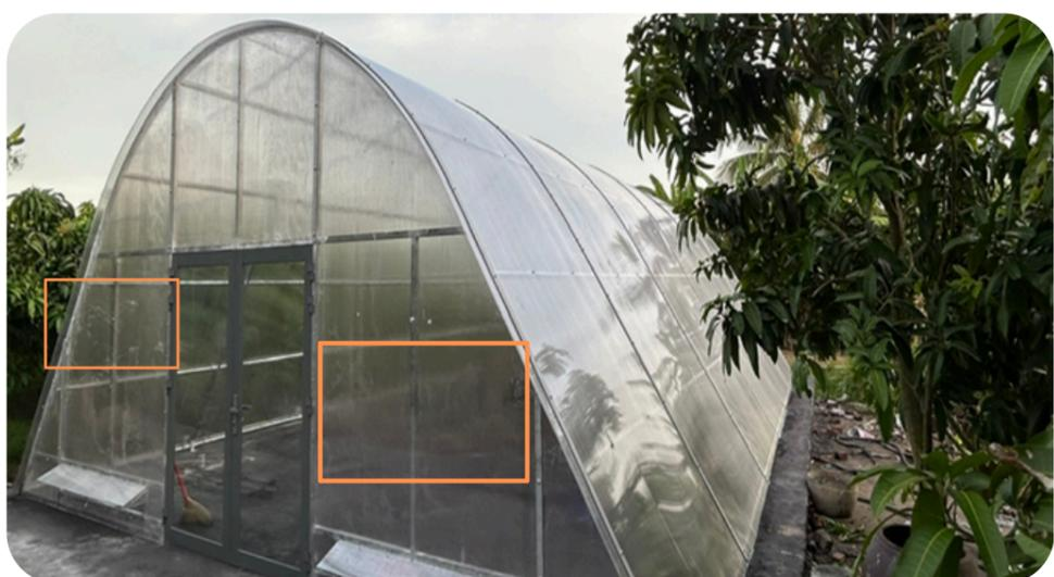
Figure 4: the air inlets placement, CDEA
